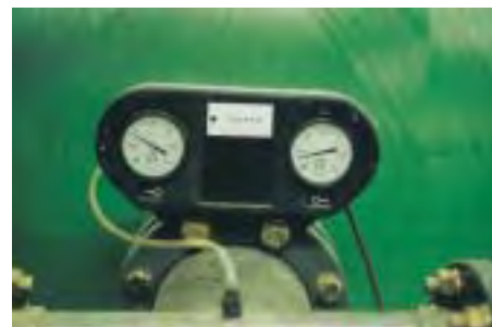
Figure 36 Pressure Differential Gauges
