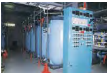
Figure 30 Plant Room with Multiple Filters
