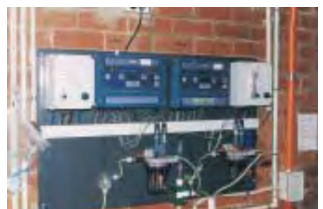
Figure 18 Pool Control Panel and Chemical Measuring Station
