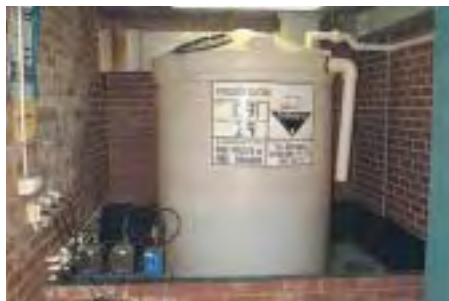
Figure 7 Bulk Sodium Hypochlorite Container in Bund
