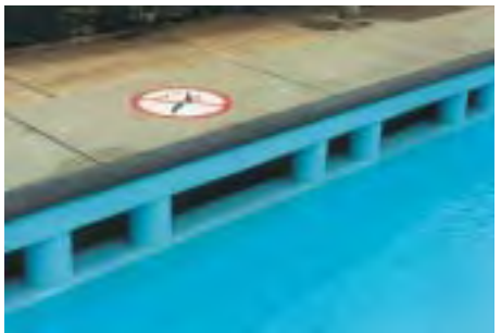
Figure 26 Overflow Channel on an Older Outdoor Pool
