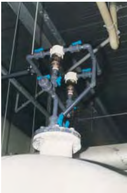
Figure 33 Filter Off-Gas Bleed and Collectors
