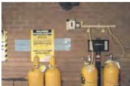
Figure 6 Chlorine Gas, Weight Scales and Regulator
