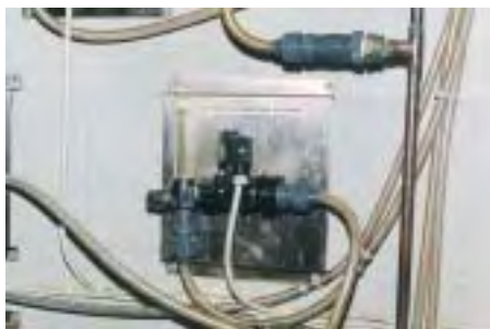
Figure 16 Carbon Dioxide Controller
