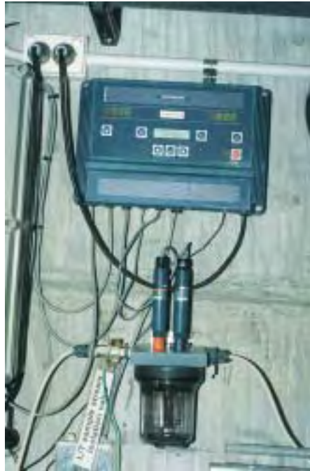
Figure 19 Chemical Sensors Installed in a Side-Stream Loop
