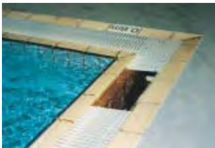
Figure 25 Wet Deck on a Modern Indoor Pool
