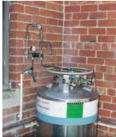
Figure 13 Carbon Dioxide Tank
