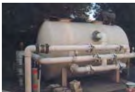
Figure 29 Medium Rate Pressure Filter for Larger Pool
