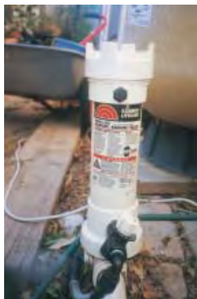
Figure 17 Erosion Canister (Erosion Feeder)
