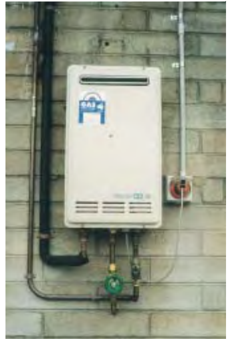
Figure 5 Instantaneous Hot Water Systems
