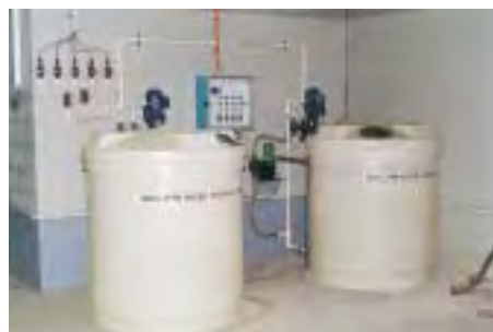
Figure 35 Dosing Tanks with Mixers for Adding Coagulant
