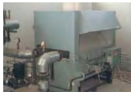
Figure 40 Heavy Duty Gas or Electric Boilers
