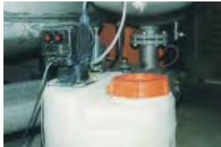
Figure 15 Metering Pump
